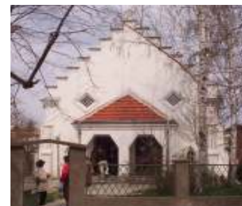
The Lom church building
